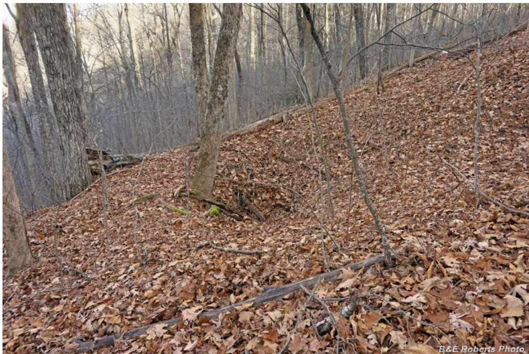
Main Pit (caved in) - Spaniard Mica Mine
